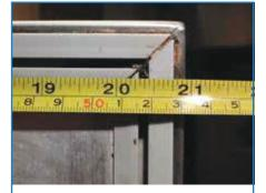
When placing your order note that the dimensions are dart to dart and we will convert your measurements to outside edge dimensions.
